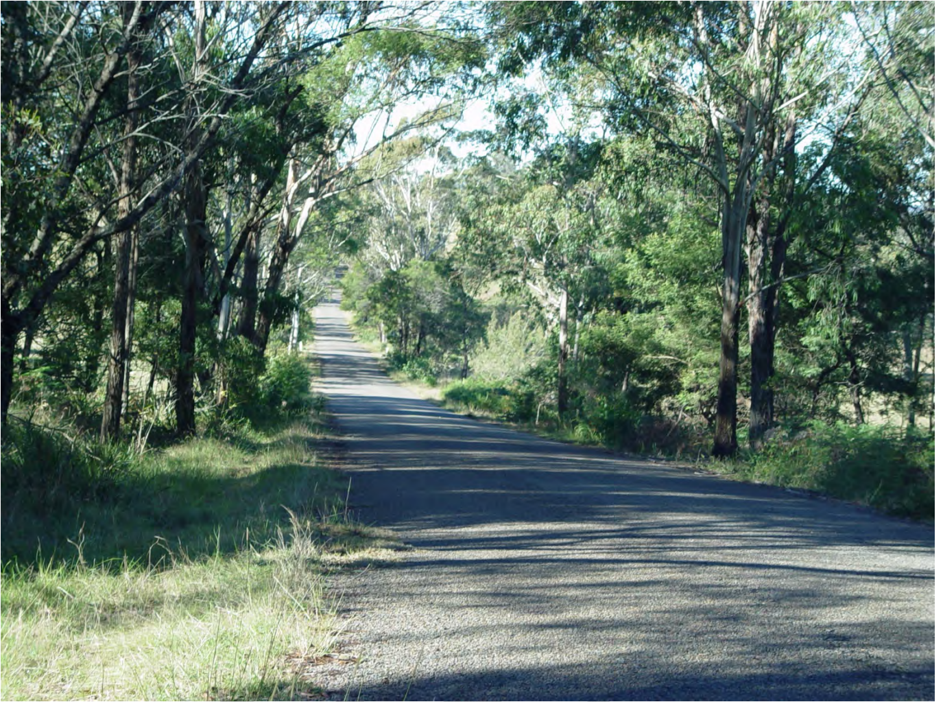
Photo 12 – Compton Park Road bitumen sealed section from Green Hills Road
