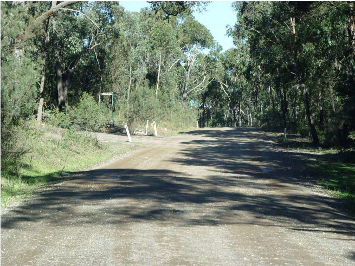
Photo 5 – Looking south (towards Berrima) along Old Mandemar Road at Compton Park Road intersection
